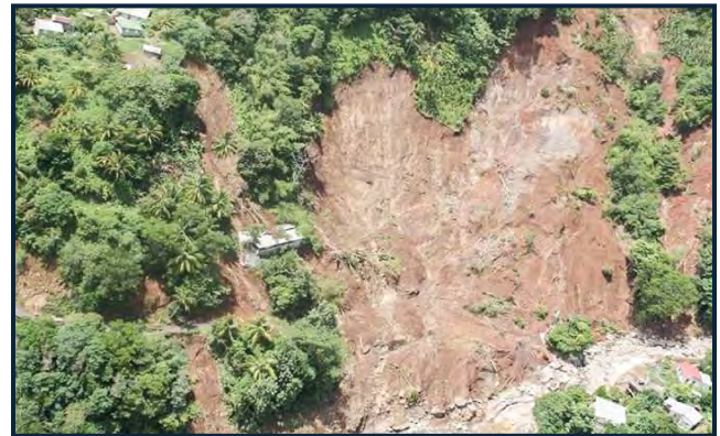
Damages from Tropical Storm Erika
