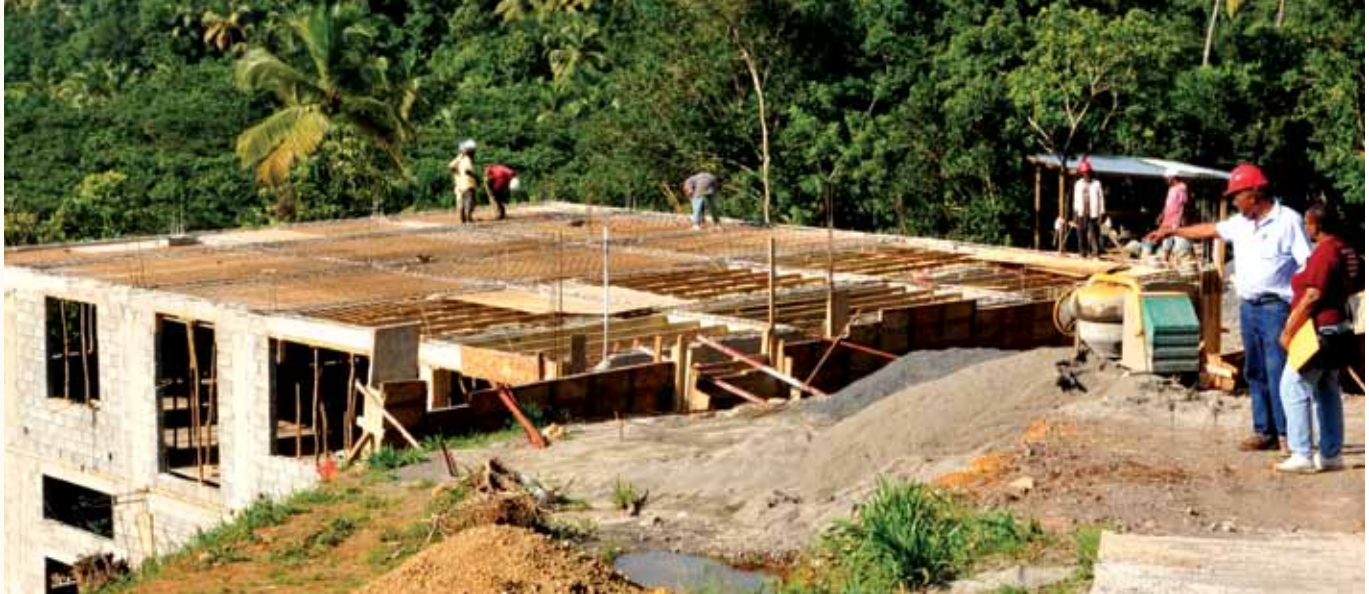
Construction of Resort and Spa, Anse De Mai
