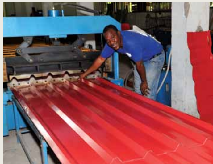
Manufacturing of Aluminum Roofing, Portsmouth
