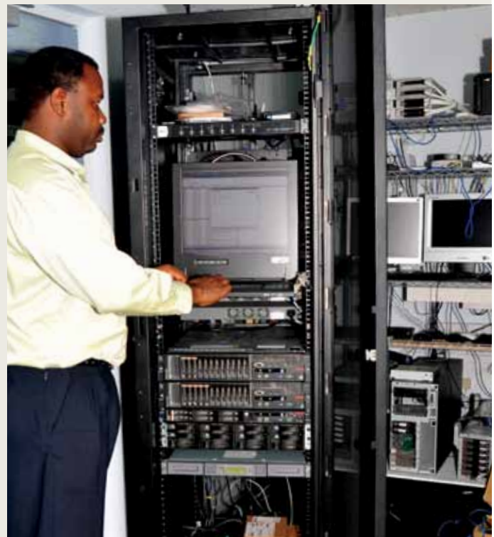
New Equipment installation, MIS Unit, AID Bank
